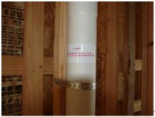
←Be sure to clearly label the soil gas ventilation pipe so it
