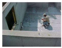
←A sheet of six mil. Polyethylene sheeting (or three mil.
