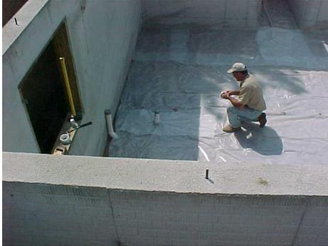
← A sheet of six mil. Polyethylene sheeting (or three mil. cross-laminated sheeting) laying on top of the gravel aggregate.
