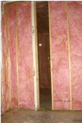
← A 3- or 4-inch diameter PVC ventilation pipe, rising vertically from the gravel bed beneath the basement floor through the attic, and out letting above the roof.
