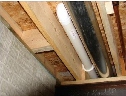
← To function without a fan, the soil gas ventilation pipe must be installed vertically (plumb); even warm air will not rise when channeled through a horizontal run of pipe like this.
