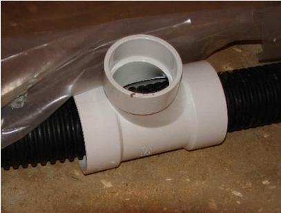
← You can also adapt the SGVS to treat a crawlspace. Soil gas is trapped beneath a sheet of 6-mil plastic (or better) membrane which is laid on the soil surface throughout the entire crawlspace. Then the membrane is attached about 12" up on the side walls.
