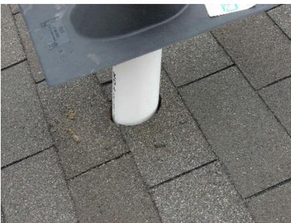
←The outlet of a passive soil gas ventilation system should penetrate the roof on the back-side of the home.
