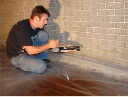
← As a best management practice, seal all joints, cracks, and openings around utility penetrations in the floor and walls below grade. Use an elastomeric sealant to provide an airtight seal.
