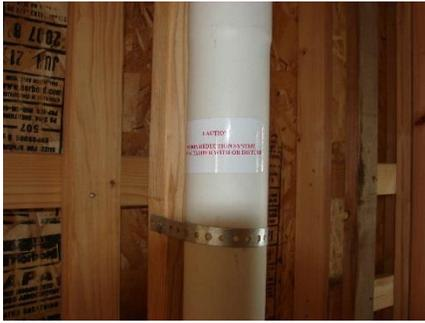
← Be sure to clearly label the soil gas ventilation pipe so it doesn't get confused with other utility systems.
