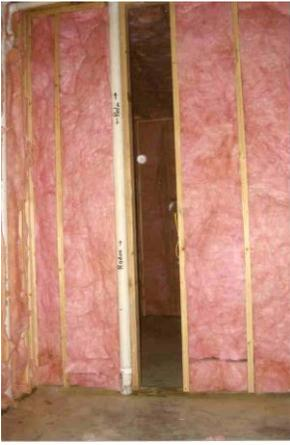
←The vertical, soil gas ventilation pipe must be installed within the conditioned floor area of the home. If the ventilation pipe is installed in an exterior wall, it will be typically too cold to function by natural convection. Most vertical ventilation pipes can be hidden within an interior wall.
